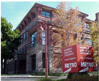
Guthrie School Building Corporate Headquarters, Wilkes-Barre, PA
